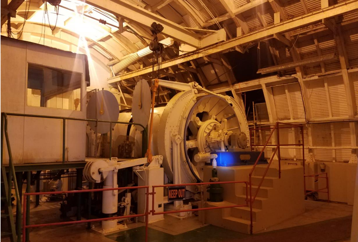
Figure 18-8 #2 Shaft Double Drum Hoist Room
