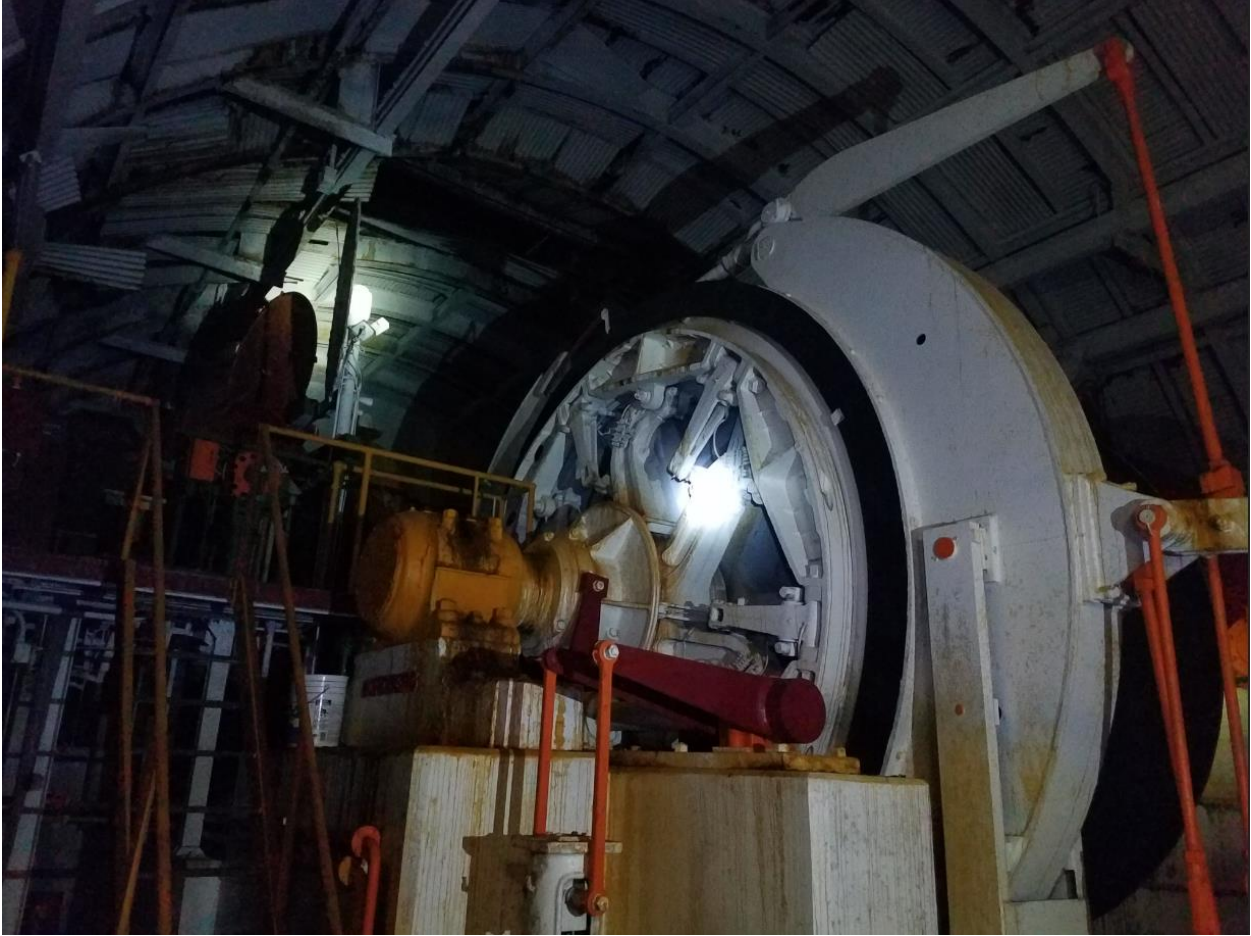
Figure 18-3 #1 Hoist and Hoist Room 9-Level
