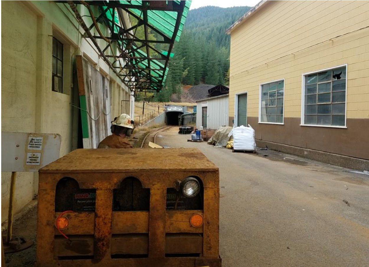
Figure 18-1 Kellogg Office Complex and Kellogg Tunnel Portal
