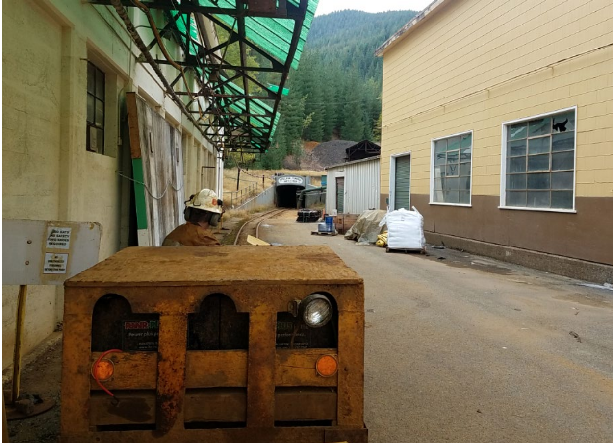
Figure 18-1 Kellogg Office Complex and Kellogg Tunnel Portal
