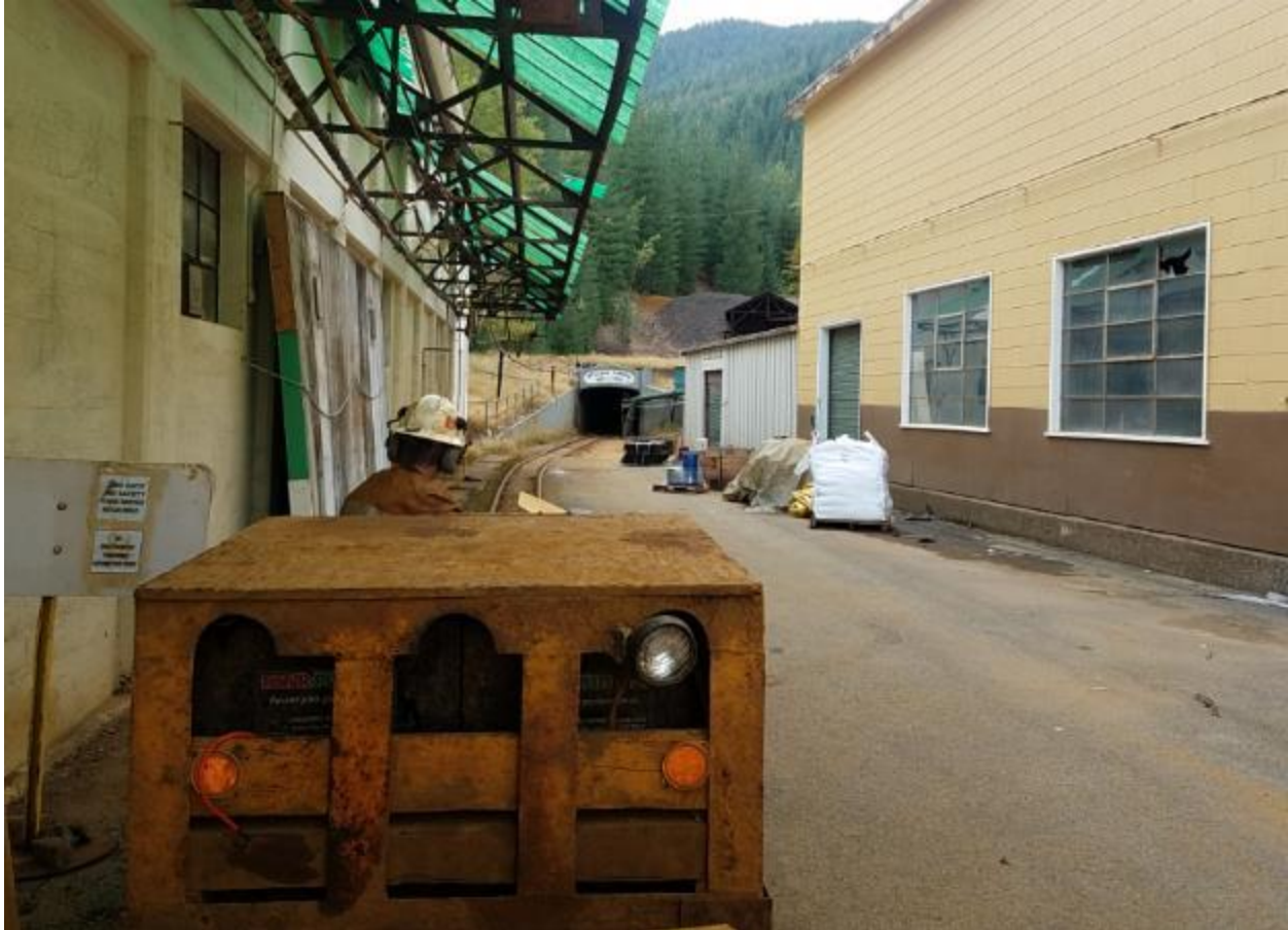
Figure 18-1 Kellogg Office Complex and Kellogg Tunnel Portal
