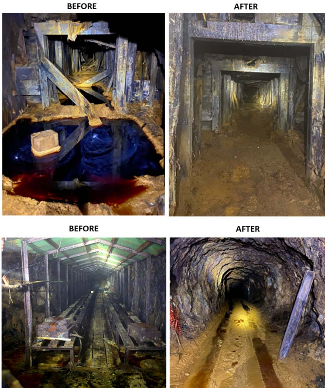
Figure 2: Before and after pictures of ground water improvements
