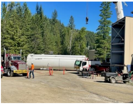
Photo 7: Lime silo being prepared for transport
