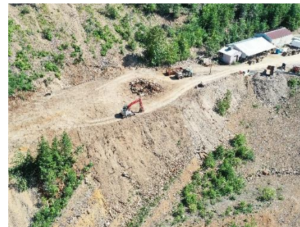
Photo 8: Wardner clean-up area
