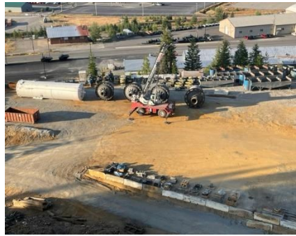
Photo 5: Balls mills, flotation cells and lime silo unloaded in Bunker Hill yard
