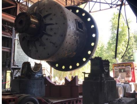
Photo 2: Ball mill hoisted by 265 ton crane
