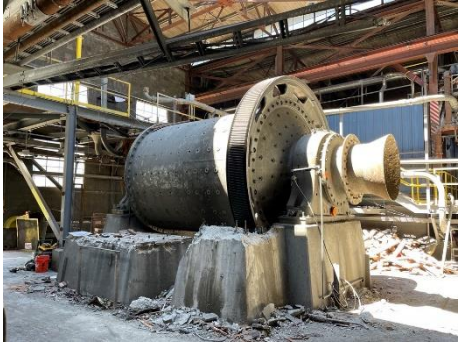
Photo 1: Regrind mill prior to transport
