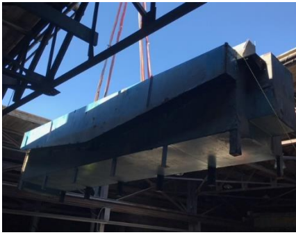
Photo 4: Flotation cell lifted through roof of Pend Oreille Mill
