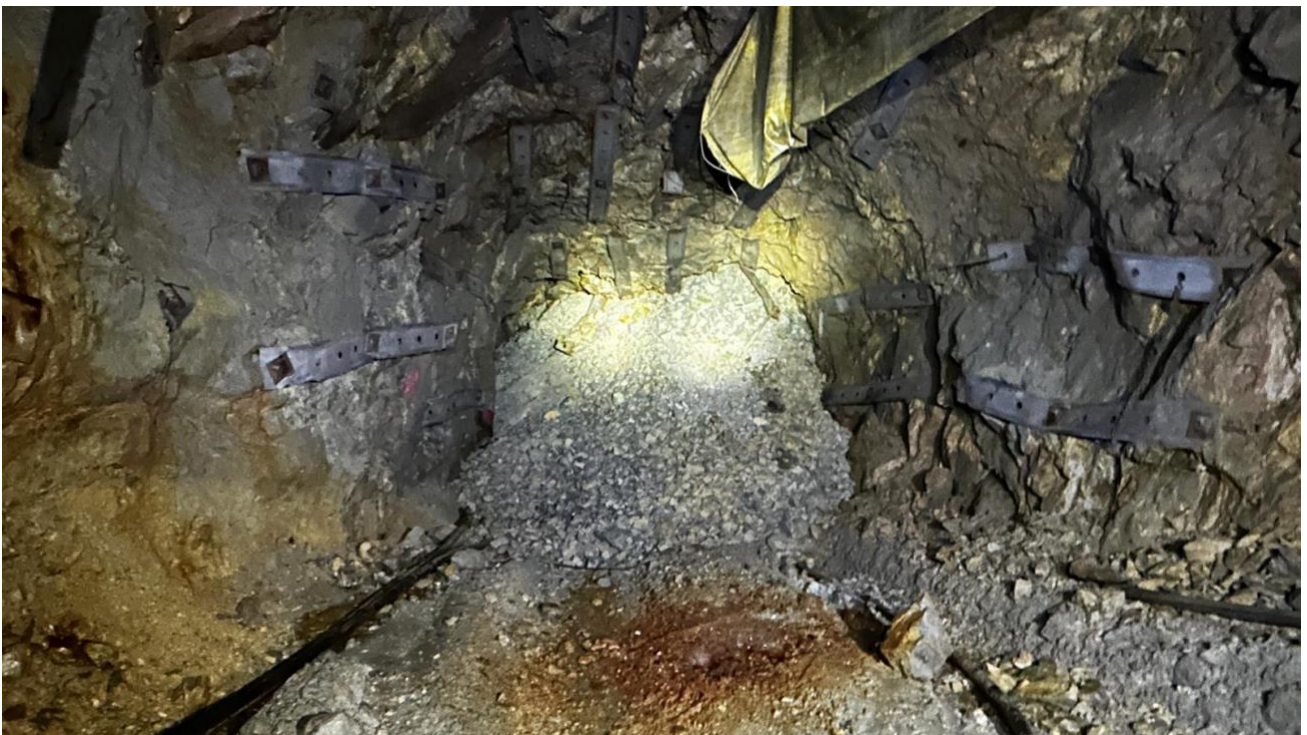
Figure 2: Bottom cut of first Underground stope at Bunker Hill FOUR YEARS WITHOUT A LOST TIME INCIDENT
