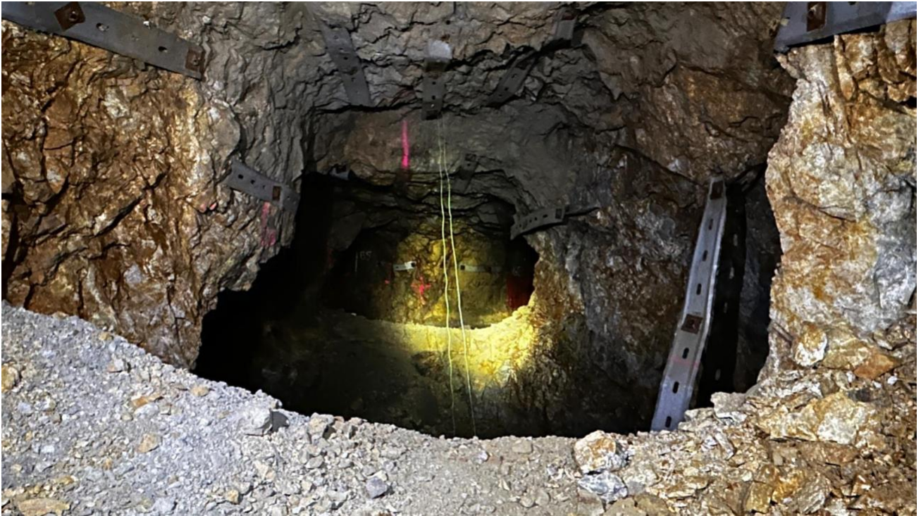
Figure 1: Top cut of first Underground stope at Bunker Hill
