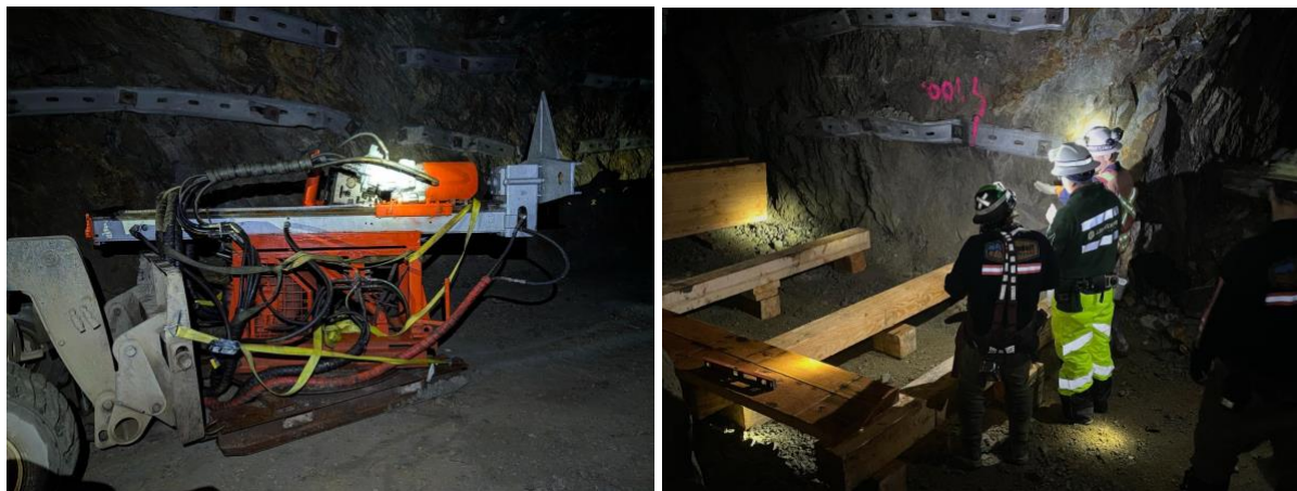
Figure 2: Underground Drill Station being prepared on 8 Level – April 13, 2026
