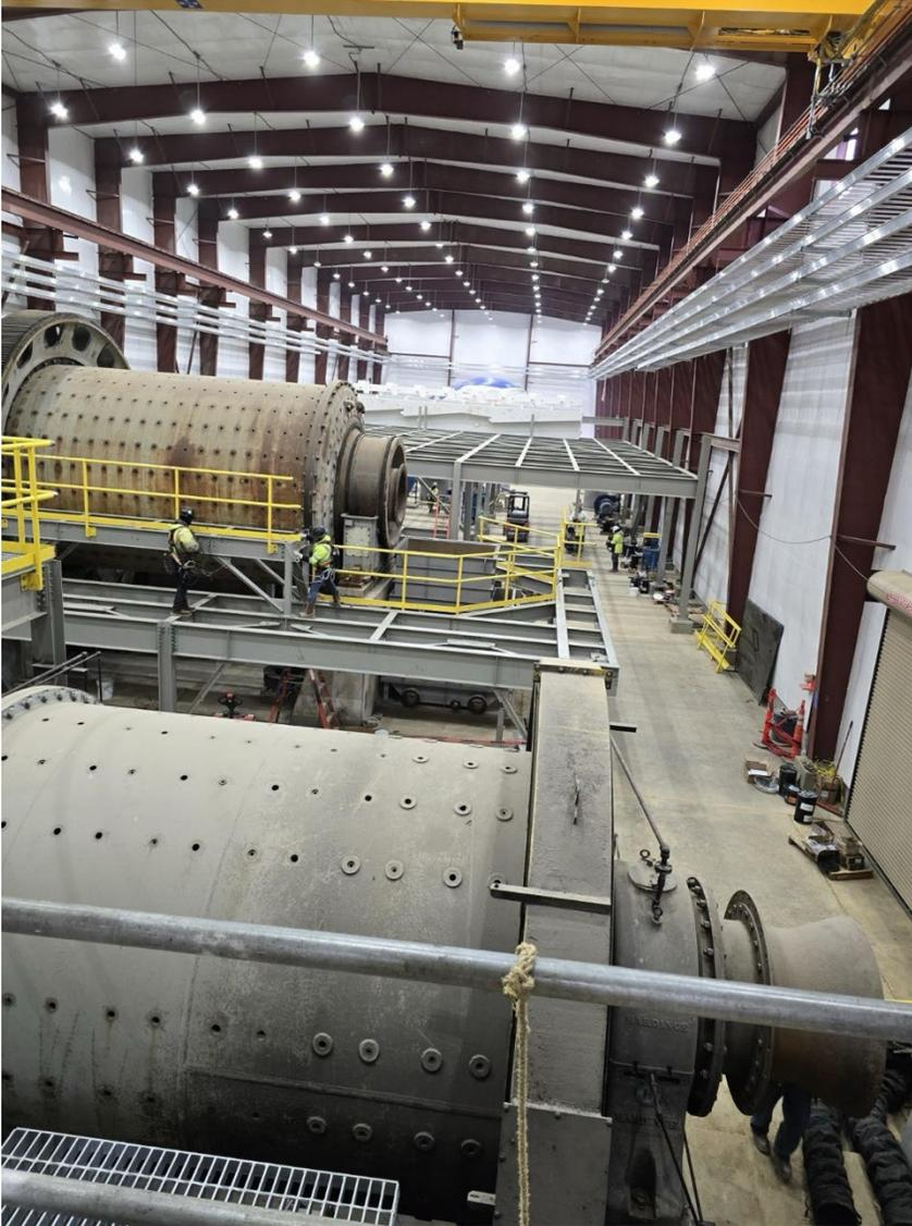
Figure 1: Installation of mezzanine access floors within the concentrator building
