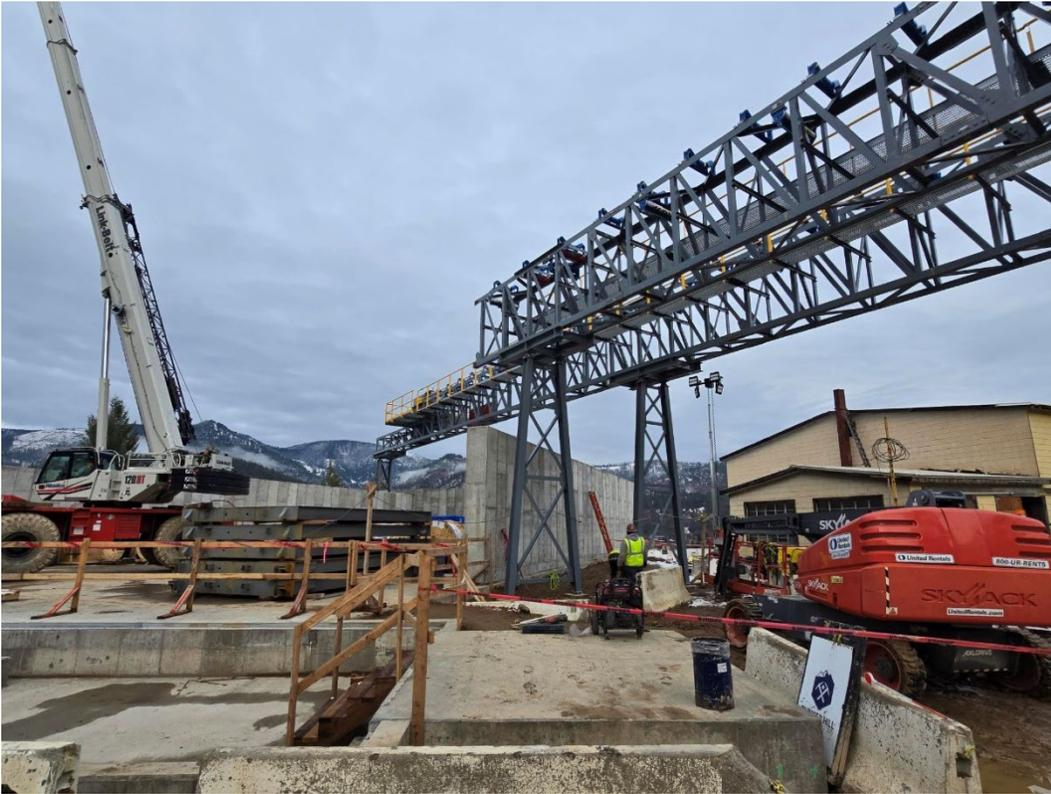
Figure 2: Conveyor infrastructure installed to feed the concentrate load-out facility
