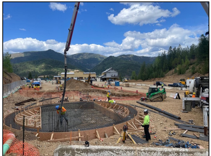
Concrete being poured on 13 May 2024 into the foundations of the Ore Bin, looking North towards the Mill Offices, Maintenance shed, and beyond into Kellogg Town and the Silver Valley
