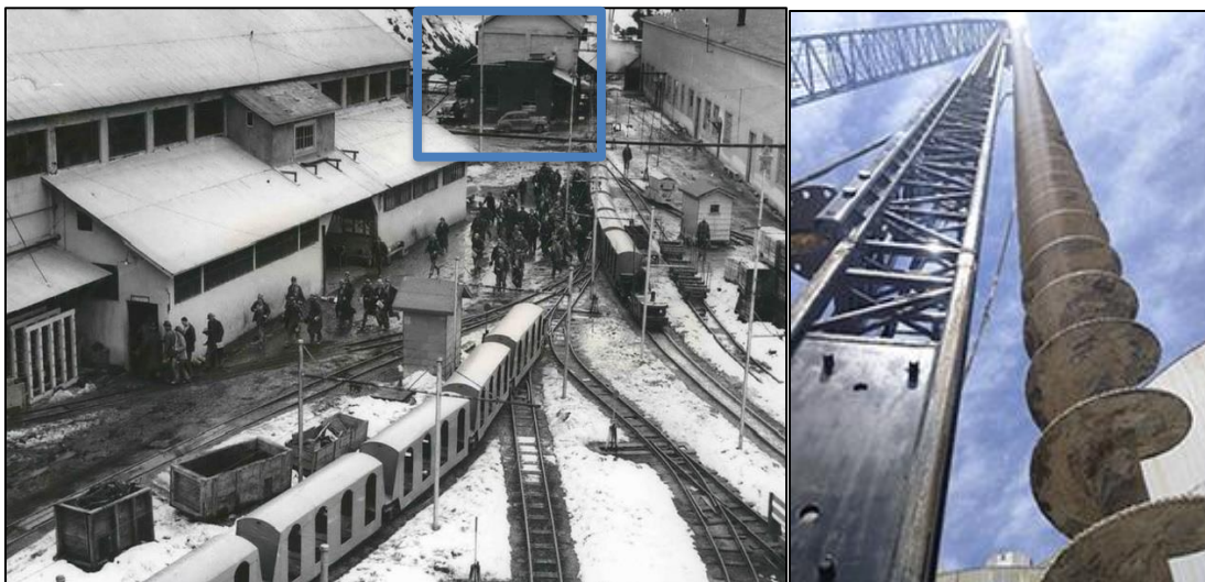
Office building in the process of being demolished shown in its historical context (L). An auger-cast pile rig operated by LFI (R)
