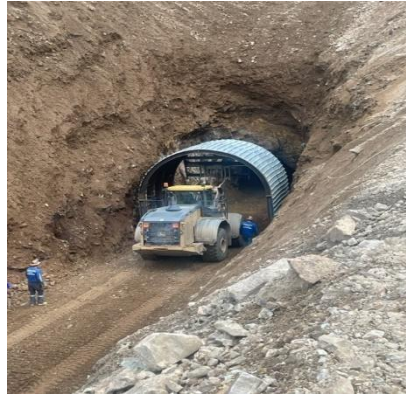
First set of steel sets being positioned.
