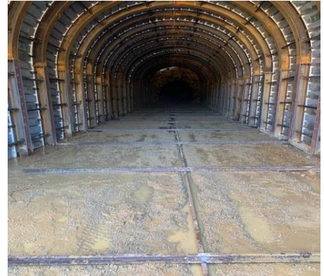
Spreaders inserted prior to burying steel sets.
