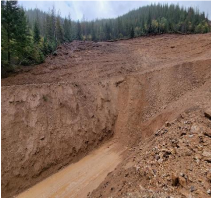
Initial earthwork in support of portal.
