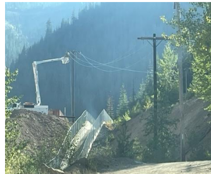
Figure 2: Wilson Construction Co. installing overhead powerlines on Bunker Hill property.
