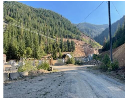
Figure 3: Overhead power installation complete at Wardner.
