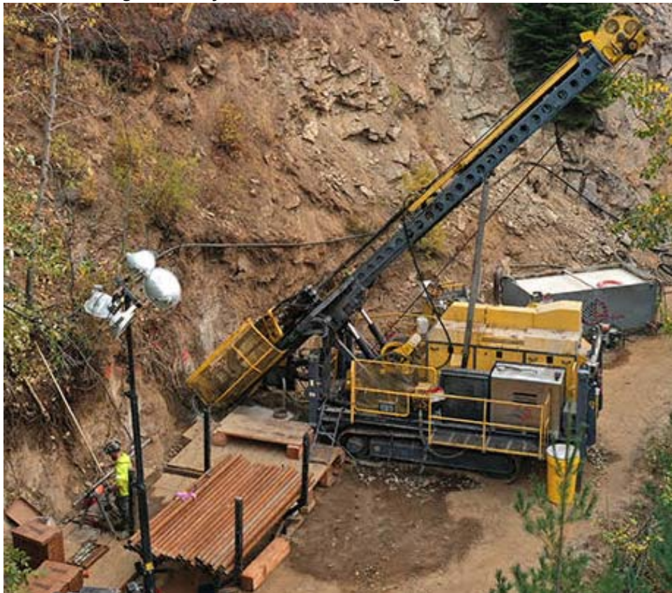
Figure 2: Surface Diamond Drill Rig at Bunker Hill Mine
