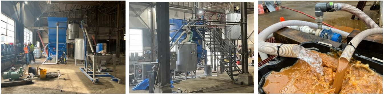
Figure 3: Photographs of Pilot Industrial Water Treatment Plant During Construction and Operation
