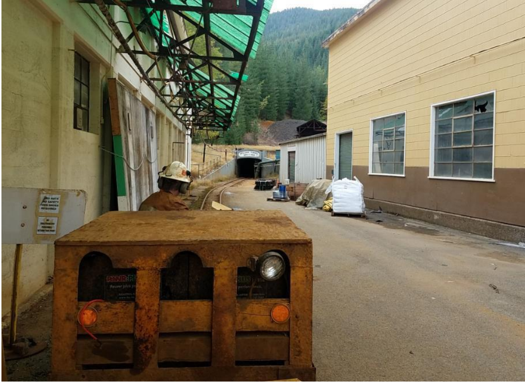
Figure 18-1 Kellogg Office Complex and Kellogg Tunnel Portal
